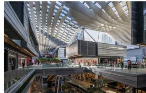
Three stories and 500,000 sf. of premier retail and restaurants make Brickell City Centre a destination of its own.
